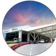
IGI AIRPORT 13 KM
